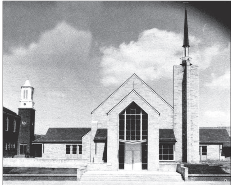
The second church completed in 1962 as it appeared on the cover of the parish's Golden Jubilee book.
