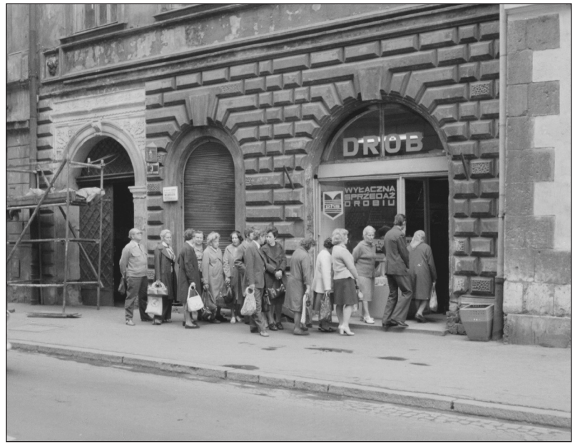
Enduring the Daily Grind. Krakow. May 23, 1976.
