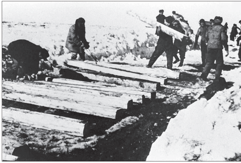
Prisoners place railroad ties on the roadbed of the North Pechora Railway, near the city of Vorkuta.
