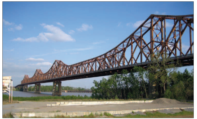
Huey P. Long Bridge
