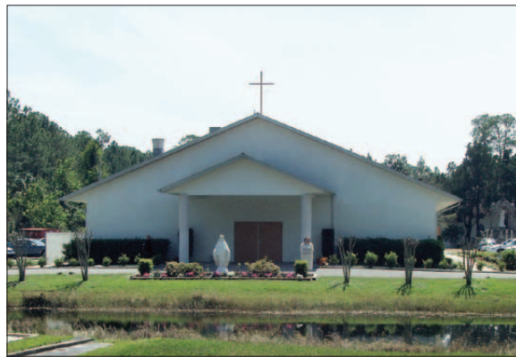
Today's St. Mary's complex as seen from the old Dixie Highway.
