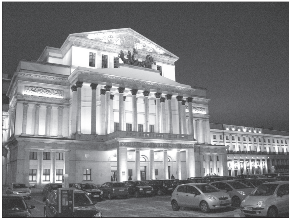
PHOTO: STAS KMIEC Warsaw's Wielki Teatr (Great Theater and National Opera House), destroyed during World War II was rebuilt, and opened in 1965, after having been closed for over twenty years.
